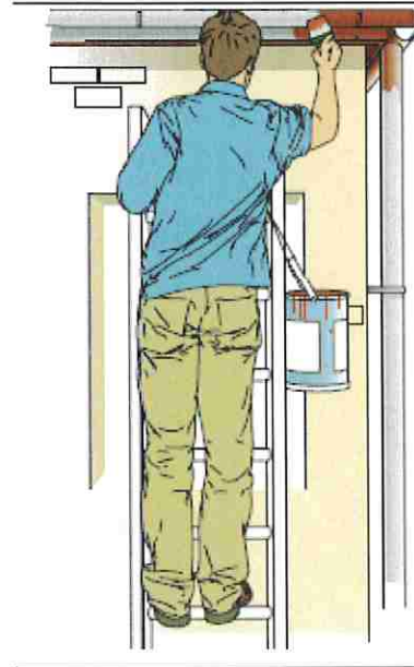
Maintaining 3 points of contact
